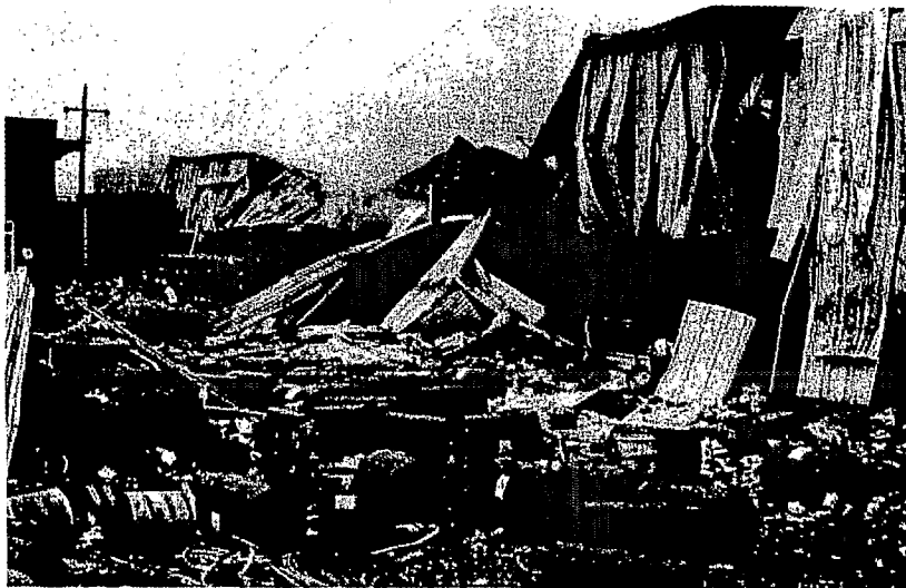
Scenes of the damage at the Shifa Pharmaceutical factory
